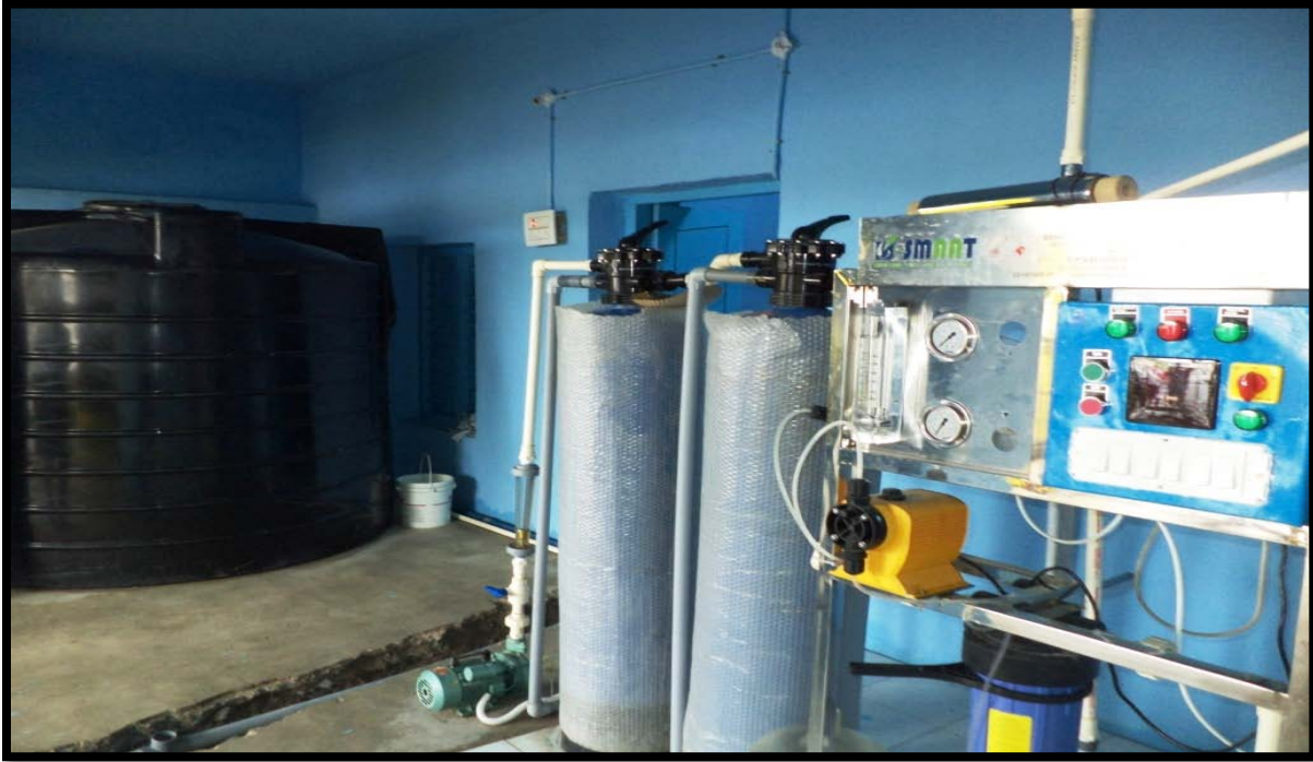
RO Water Plant Provided in Srinagar village
