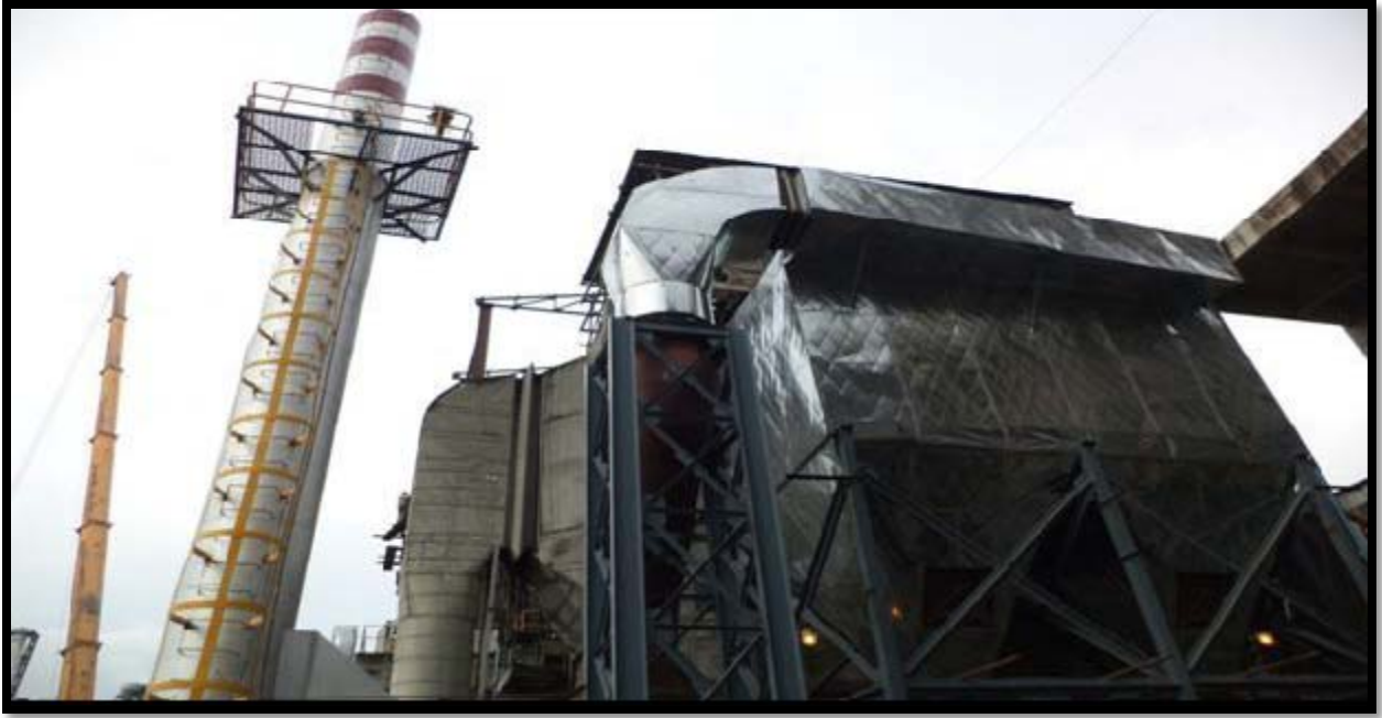
Cement Mill-2 Bag filter
