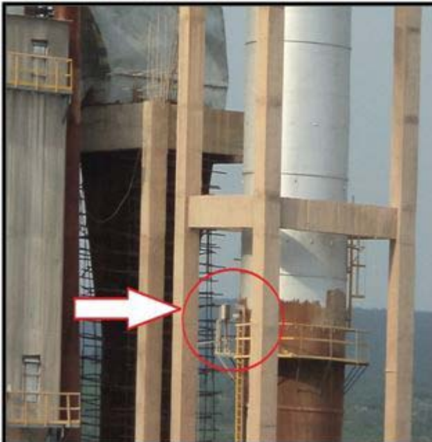
Continuous Emission monitoring Analyzer on Coal mill stack
