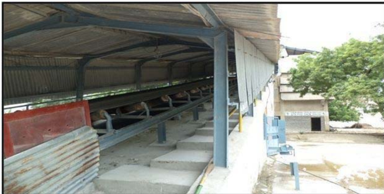
Covered belt conveyors
