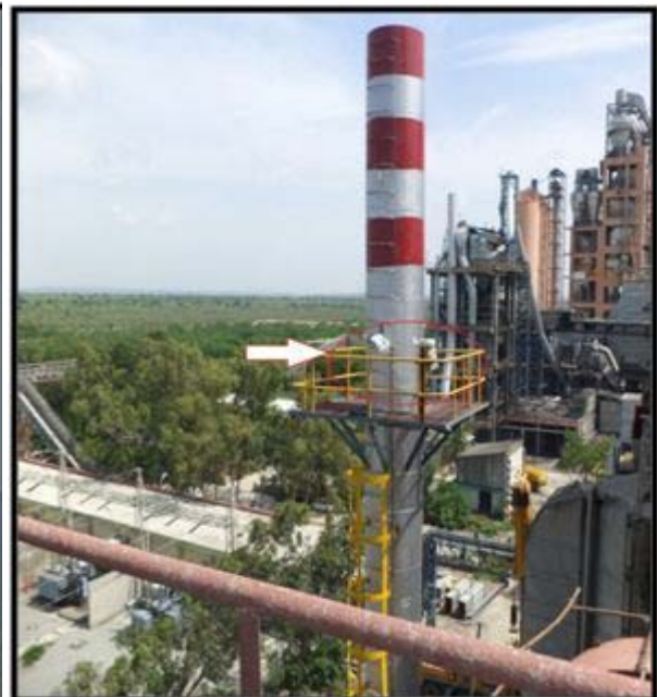
CEMS Analyzer on the Cement Mill-2 Stack
