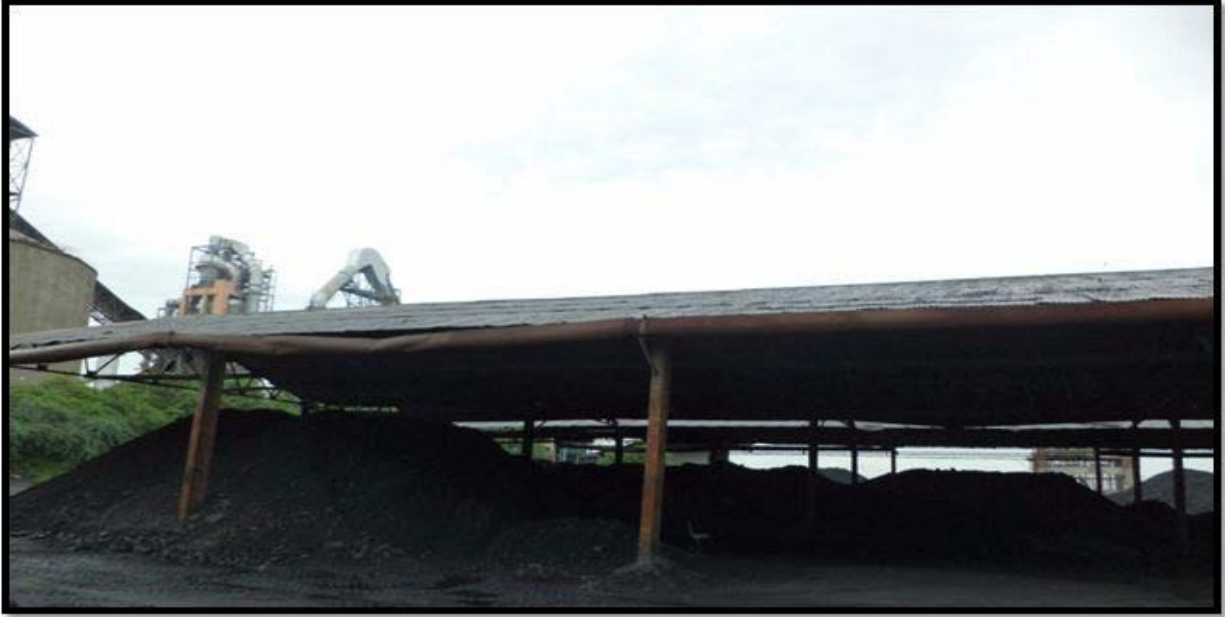
Covered Coal yard
