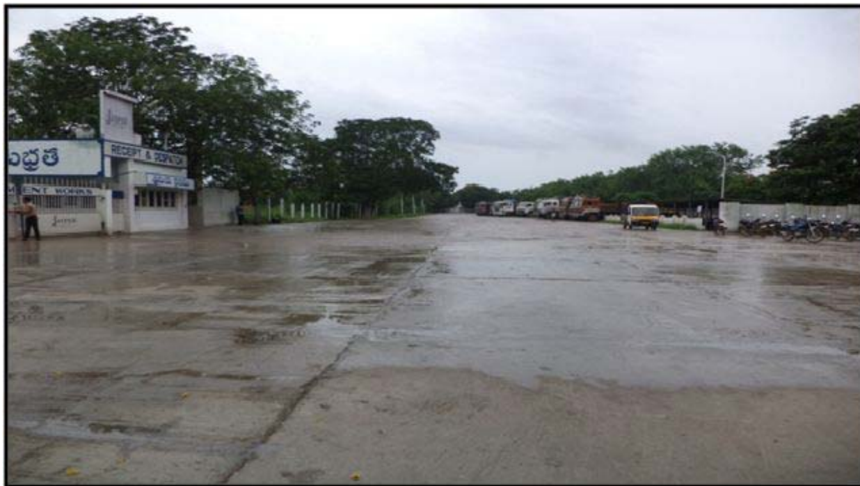
Concreted roads provided and maintained
