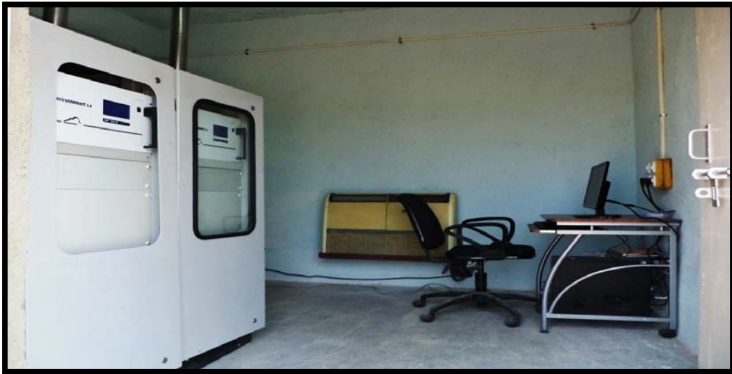
CAAQMS Station-3 installed at Mines area
