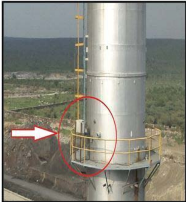
Cooler ESP Stack
